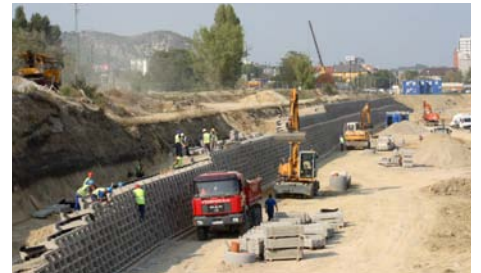
Vehicle depot is under construction
