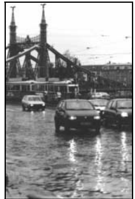
Damaged block pavement in Bartók Béla út
