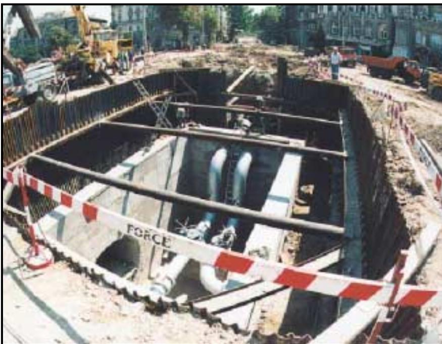
*Szent Gellért tér – construction of the shaft for district heating*
