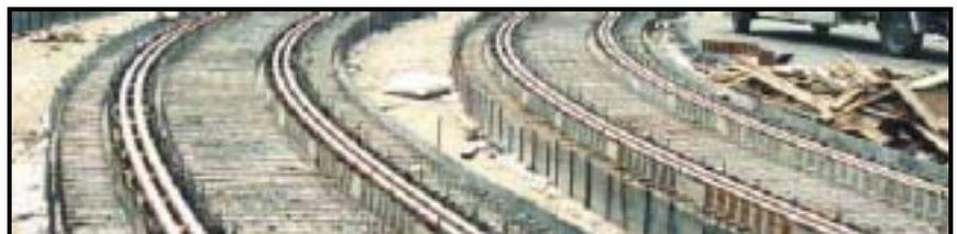
Szent Gellért tér – construction of a special track section in small arc
